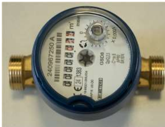
Illustration 2 Photograph showing the water meter register and dials.
